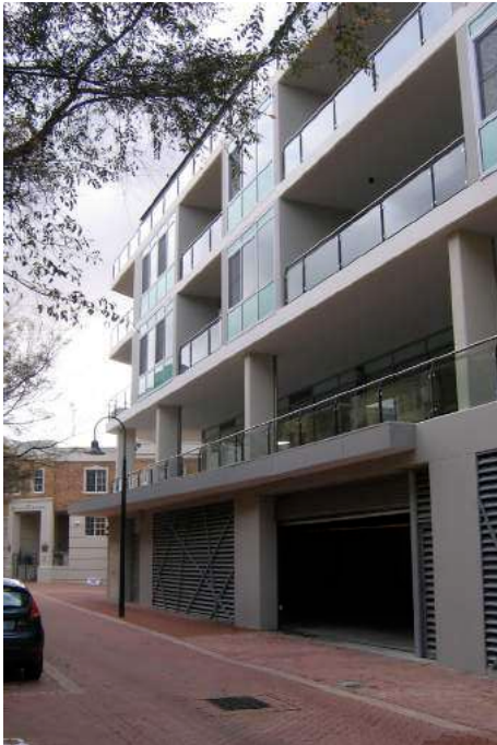
Carpark screening and consistent hardscape finish.
