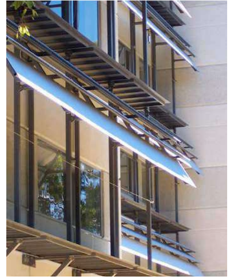
Adjustable shading devices can seasonally adapt.
