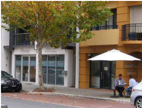
Multiple entries and apertures at ground level.
