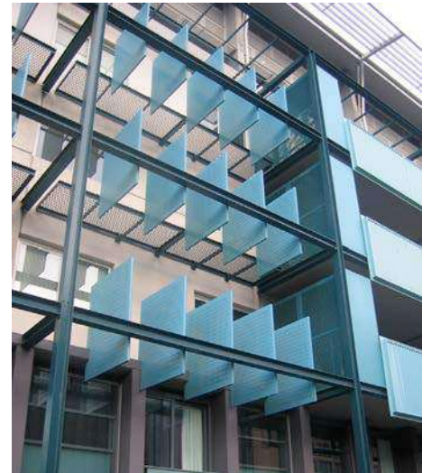
Solar shading devices provide an opportunity to enhance the character of the building.
