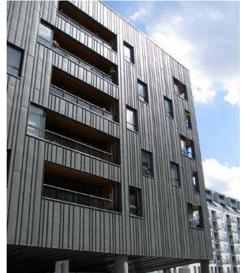
Facades designed to address local environmental conditions.
