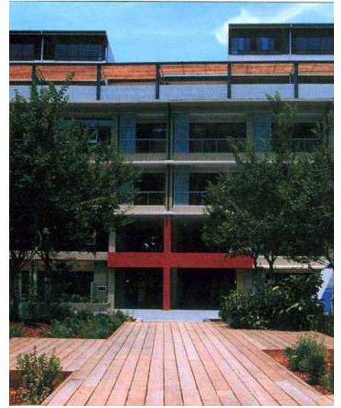
Visually highlighted building entrance.
