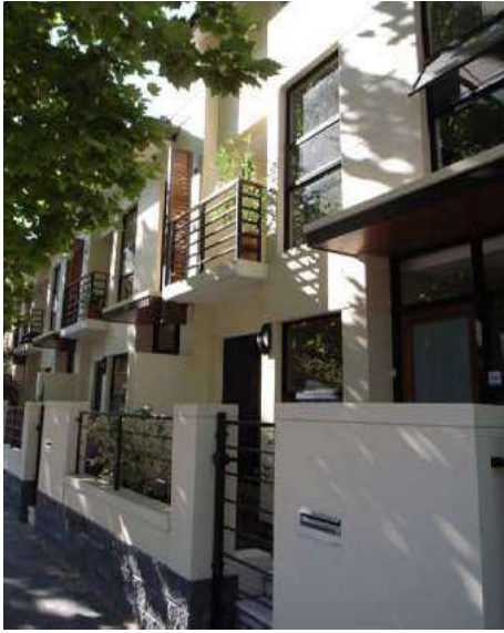
Visually permeable front fencing.
