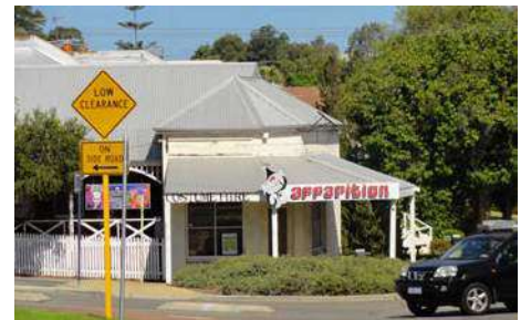
Posted awnings and traditional architecture on Shenton Avenue..
