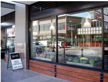
Retail and commercial frontages are encouraged to incorporate stall risers, sills glazing and fascia.
