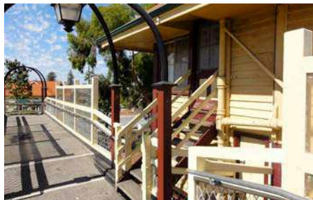
The site enjoys proximity to Claremont train station and heritage buildings.
