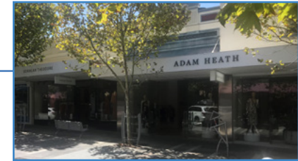
Existing character retail within the Bay View Terrace mall area.
