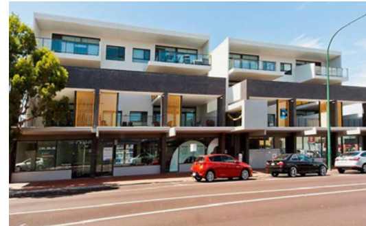
Image: Building height provisions in the PSP will achieve specific interface outcomes where appropriate.
