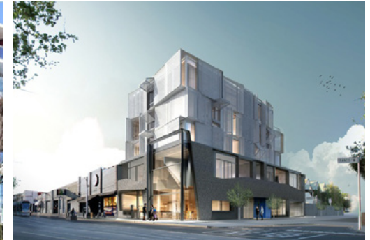
Image: Podium height maximum of two storey to achieve a 'human-scale' at the public realm edge (5 storey building)
