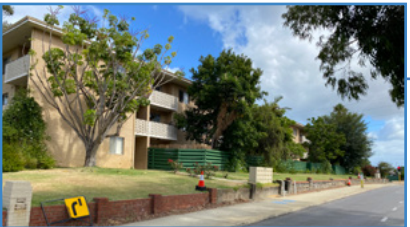
Existing higher density residential along Stirling Road.
