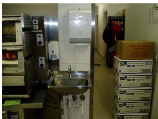
Picture 9 & 10: Hands free operated hand wash basin with paper towel and liquid soap dispenser.
