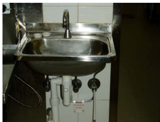
Picture 9 & 10: Hands free operated hand wash basin with paper towel and liquid soap dispenser.
