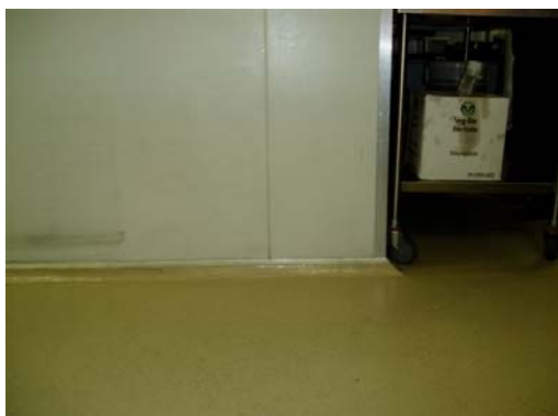
Picture 5: Epoxy coving on a coolroom floor
