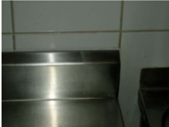
Picture 11: Sealing bench tops to wall.
