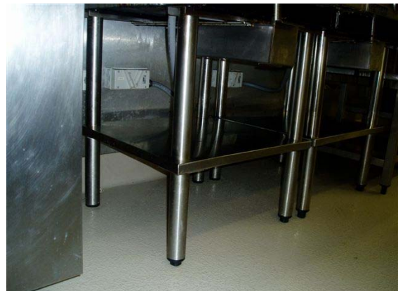
Picture 13 &14: Equipment elevated 150mm to permit cleaning underneath.
