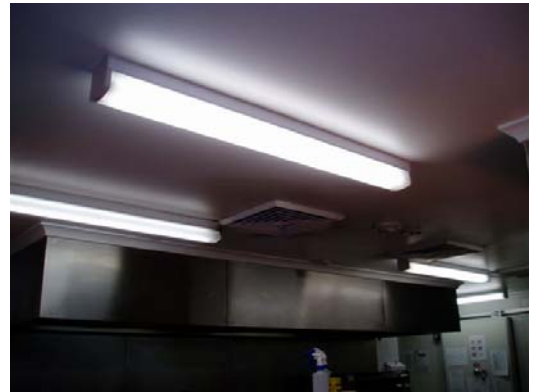
Picture 4: Light fitting flush to ceiling
