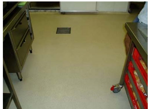
Picture 2: Floor waste
