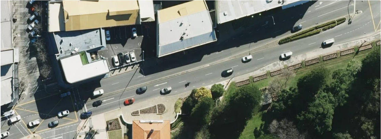
Figure 7-14 Existing bus embayment adjacent to the Town of Claremont offices
